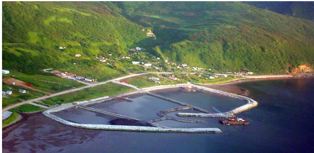
Photo 3: Aerial view of Chignik small boat harbor under construction by the Corps of Engineers; scheduled for completion Dec. 2008, summer 2003.
